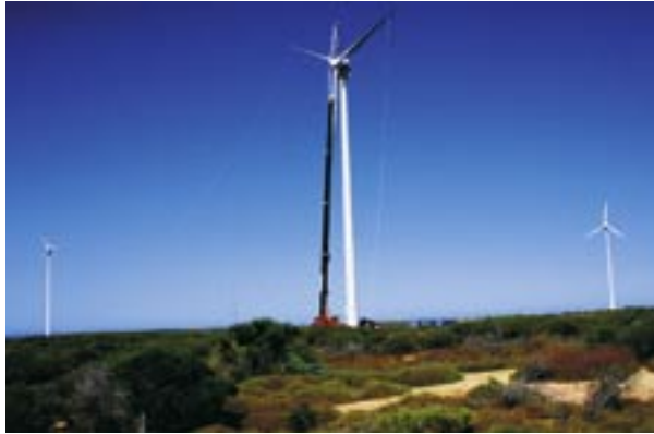
The wind farm at Denham during construction.
