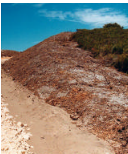
Plate 2: Well mulched batter at Chainage 1375
