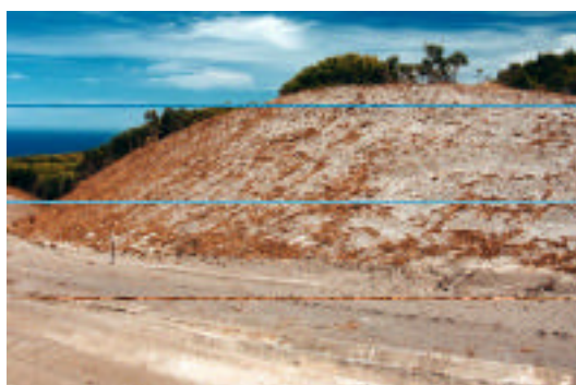
Plate 3: Partially exposed batter at Chainage 2000
