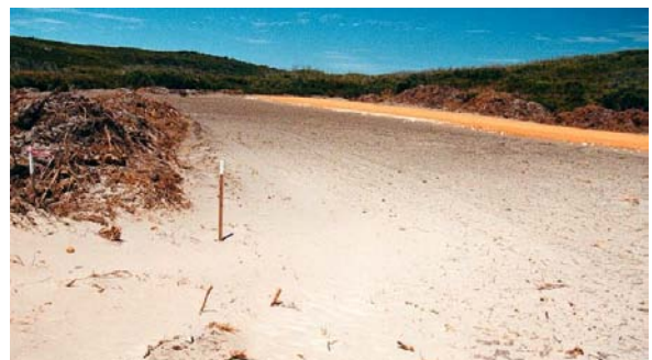
Plate 4: Turbine pad showing stockpiled topsoil and mulch
